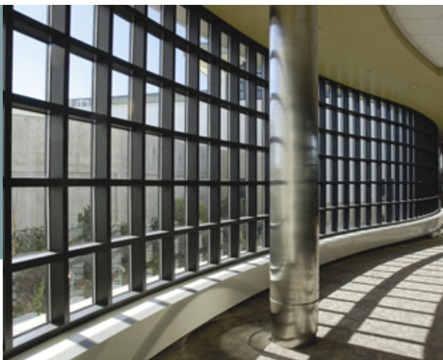
The anodizing process enhances the protective and aesthetic characteristics of aluminum with a transparent color effect that accentuates the look of the base metal. Facing page: Copper anodize window unit; photo courtesy of Marvin Window and Door. Left: Commercial-building application of bronze anodize; photo courtesy of Tubelite Inc.
