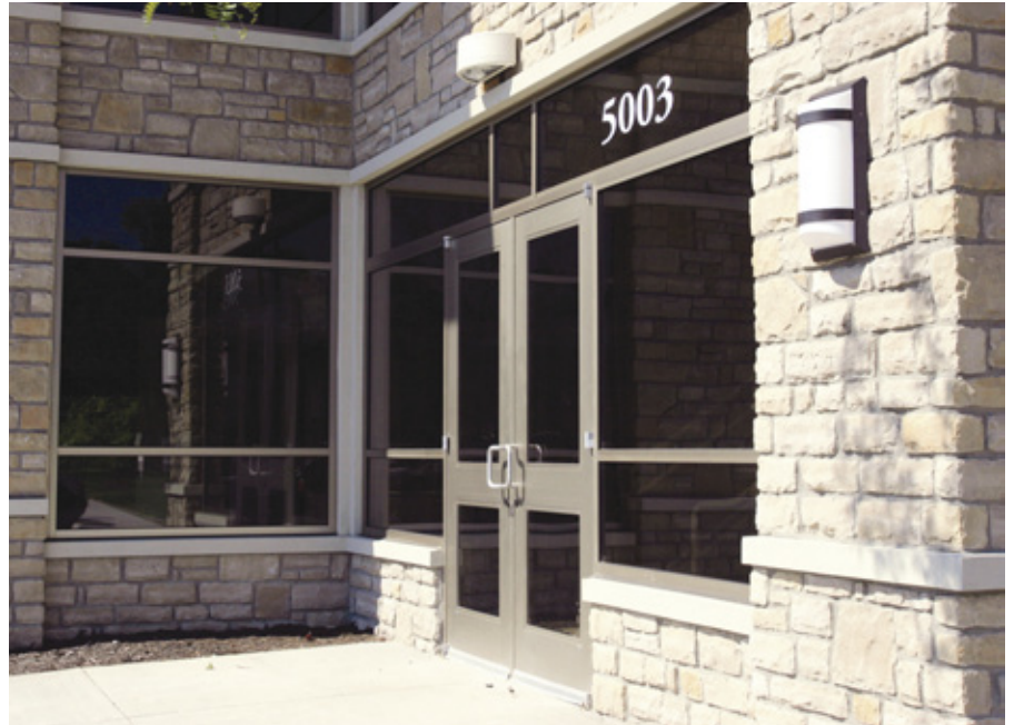
In building construction applications, anodized aluminum can be found throughout a structure's framing, in windows, doors, skylights, curtain walls, and entrances. Photo courtesy of Tubelite Inc.
